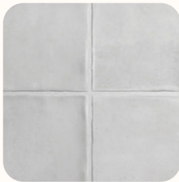
Bathroom Floor Tiles to Architect's Specification
